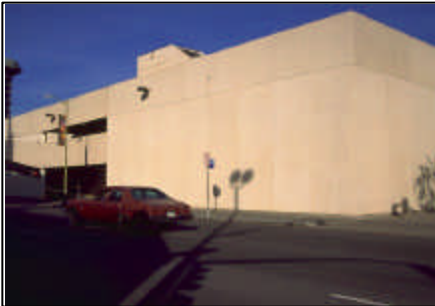
Blank walls on the ground floor are unattractive, uninviting, and are not human scale.
