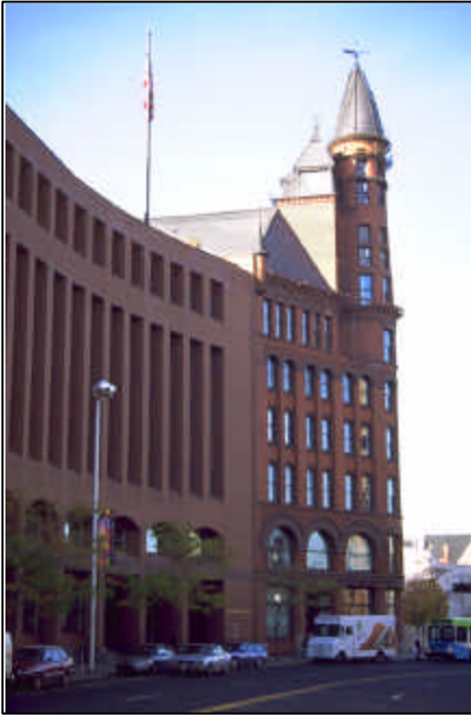
Matching cornice lines of new buildings to the traditional street façade helps to maintain an architectural continuity..
