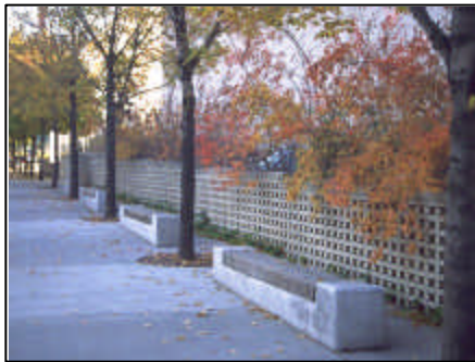
Decorative walls with landscaped amenities can screen unattractive surface parking lots from public walkways.
