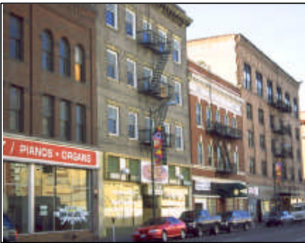
The retrofit to this historic building covers fine architectural details that could have been preserved and emphasized .
