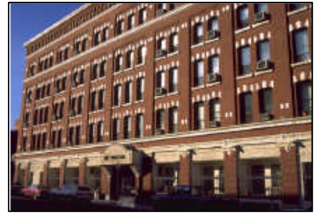
Horizontal rhythms are reinforced with similar alignments of floorlines, windowsills, cornices, and rooflines.
